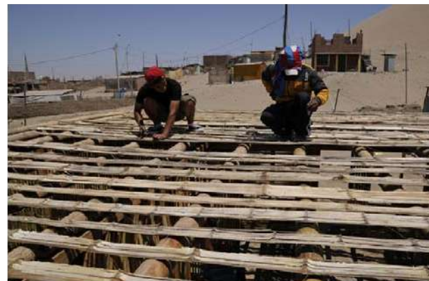
Roof composed by bamboo, reeds and clay
