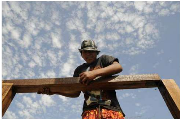
Wooden columns and beams in houses
