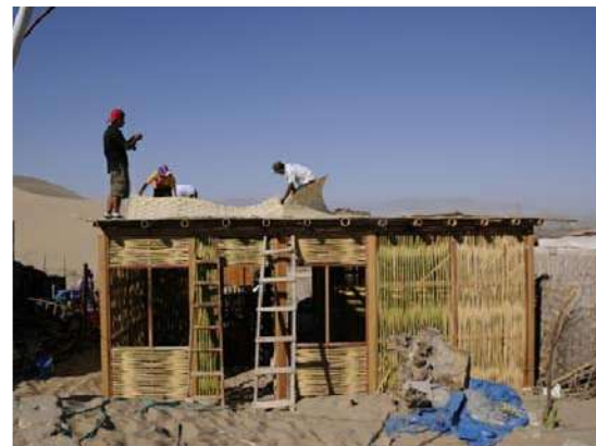
Roof composed by bamboo, reeds and clay
