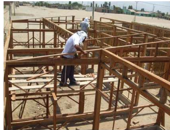
Wooden columns and beams in nursery school
