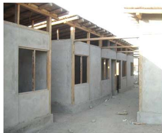
Thin layer of cement on the walls
