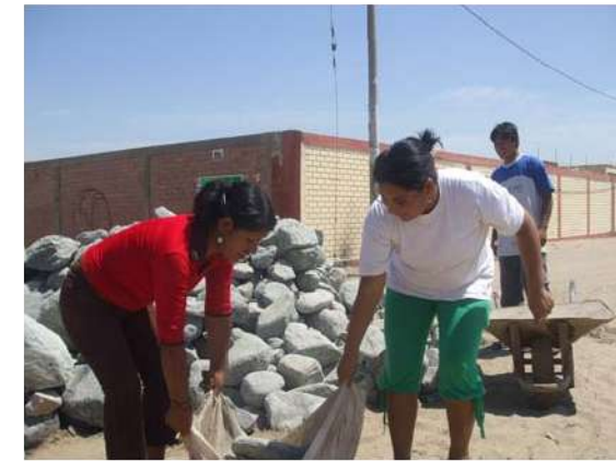
Women also supported in construction process
