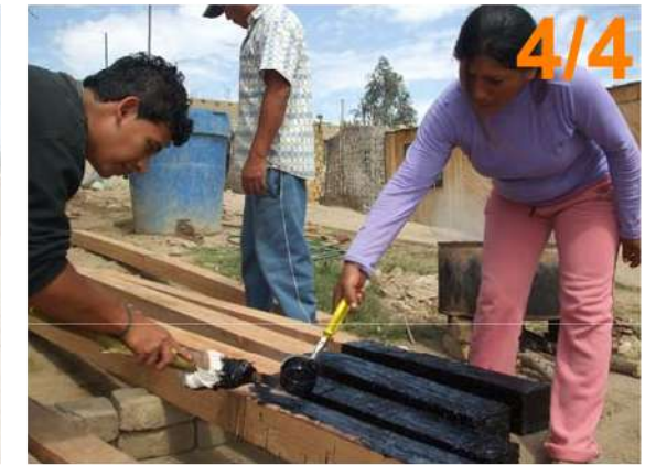
Wooden structure was protected against concrete moisture
